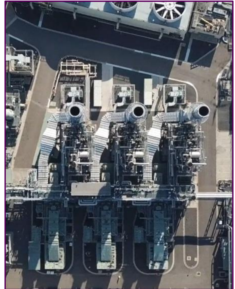
Smithfield Open Cycle Gas Turbine, NSW
