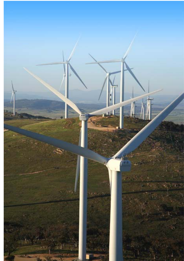
Capital Wind Farm, NSW
