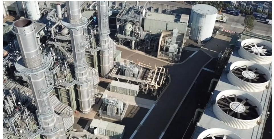
Smithfield Open Cycle Gas Turbine, NSW
