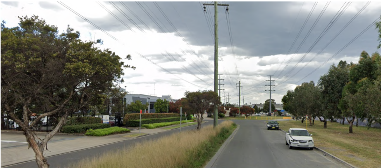
Figure 2-1 Herbert Place, facing east
