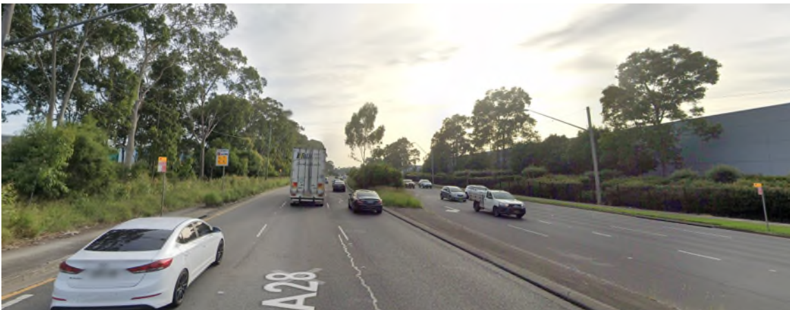
Figure 2-2 Cumberland Highway, facing north
