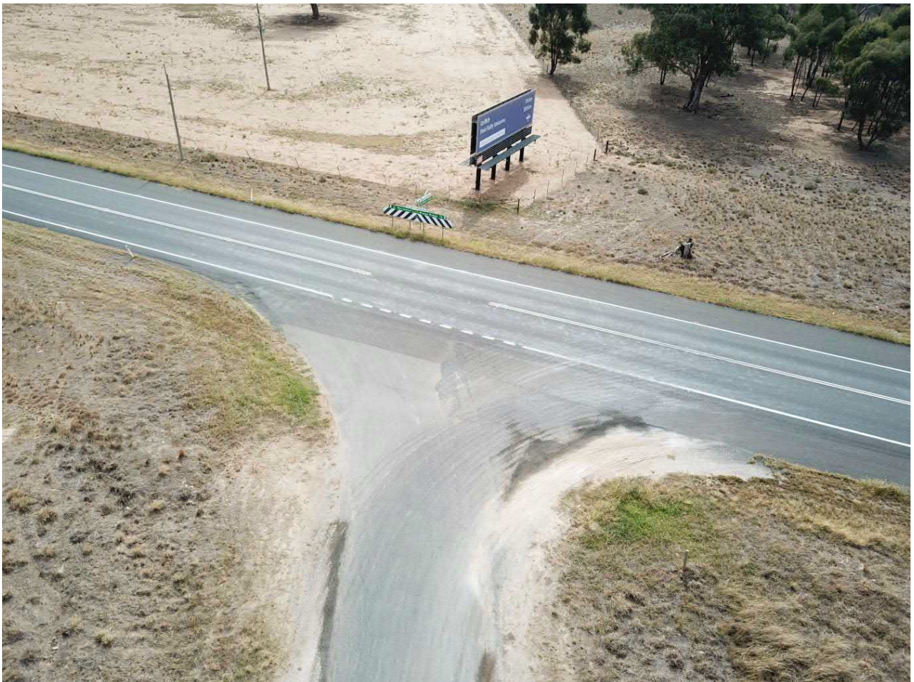
Figure 2-1: Intersection at Sturt Highway and Sandigo road looking north
