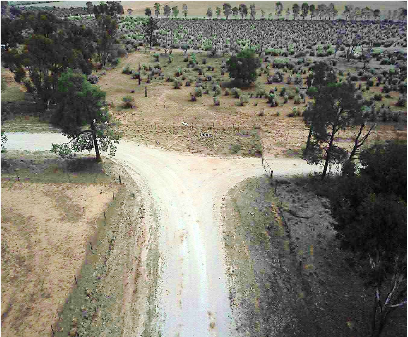
Figure 2-3: Approximate location of proposed site entrance at Muntz Road looking west
