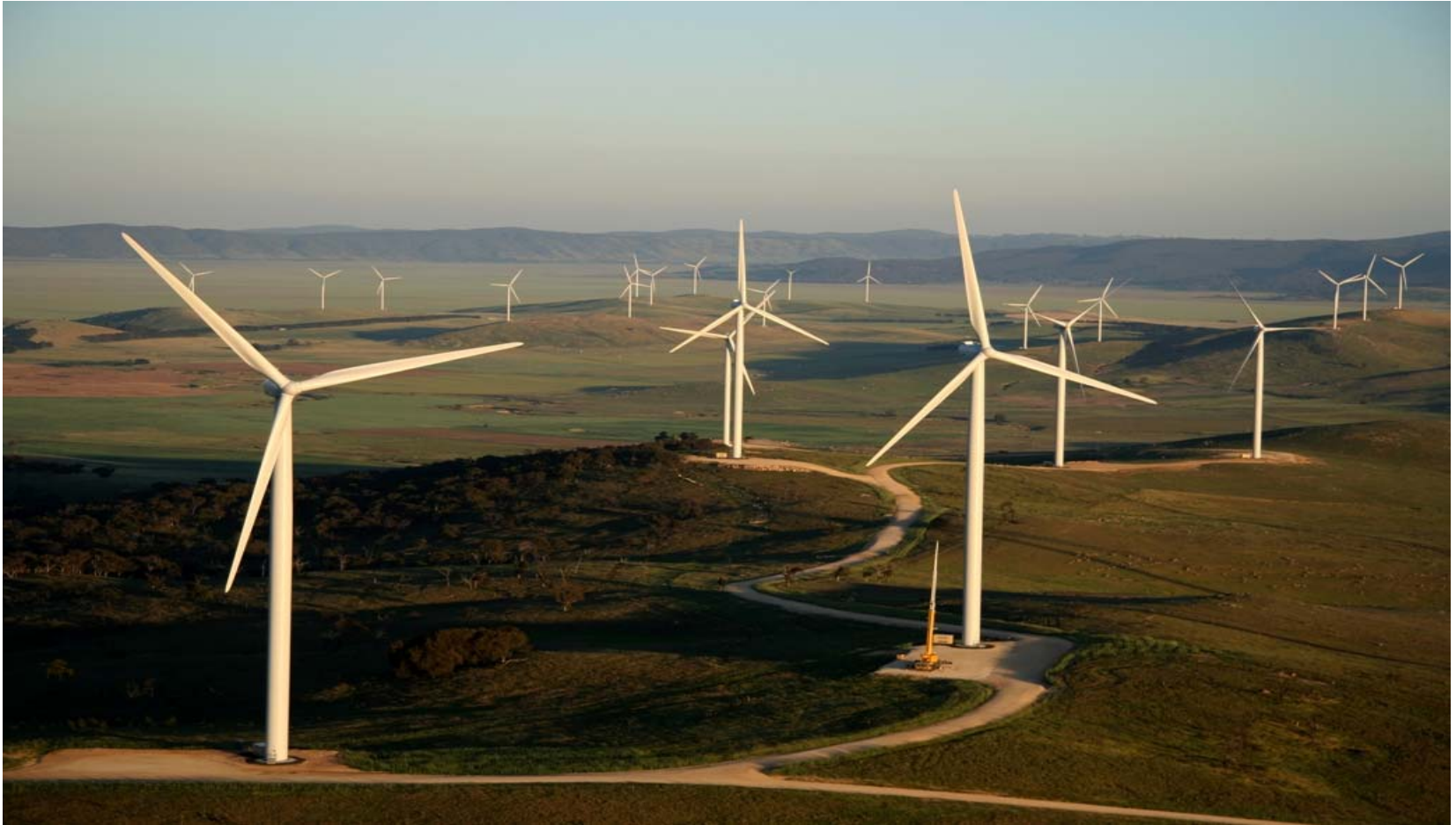
Capital Wind Farm, NSW, Australia
