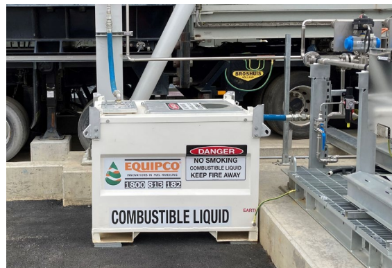
Figure 17: Turbine Fuel/Water Purge Collection Bins
