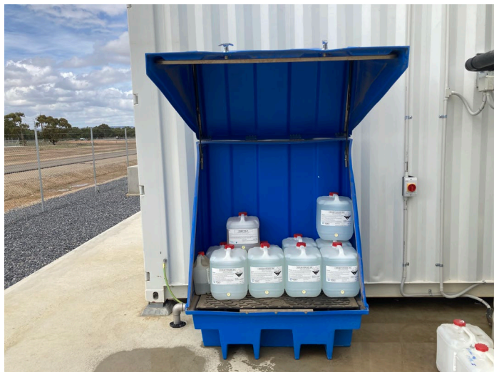
Figure 16: Chemical Storage in Mobile Bunds
