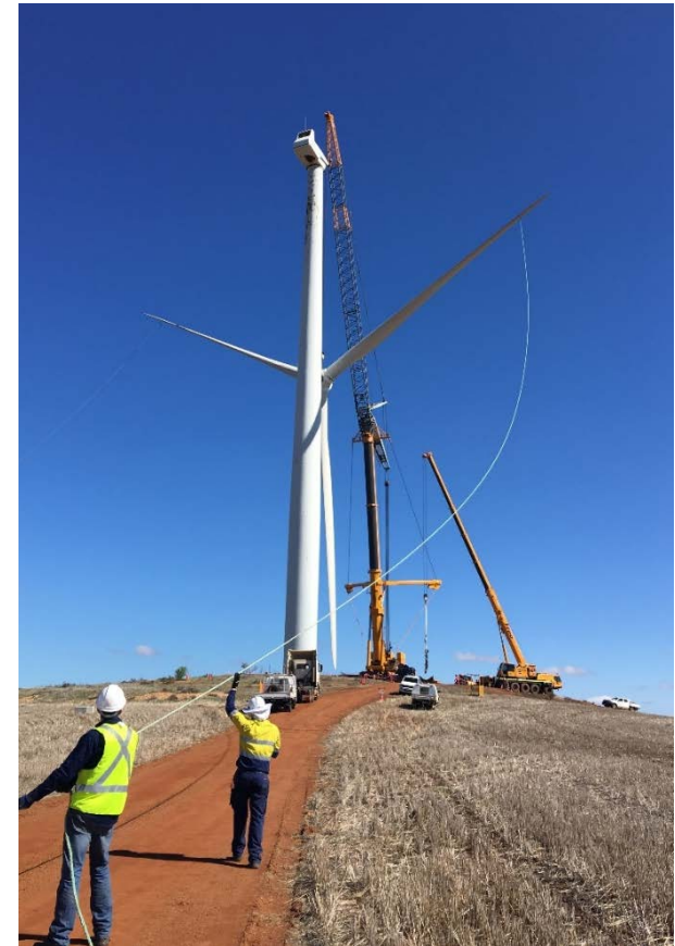
Crane lift, Alinta wind farm, April 2016
