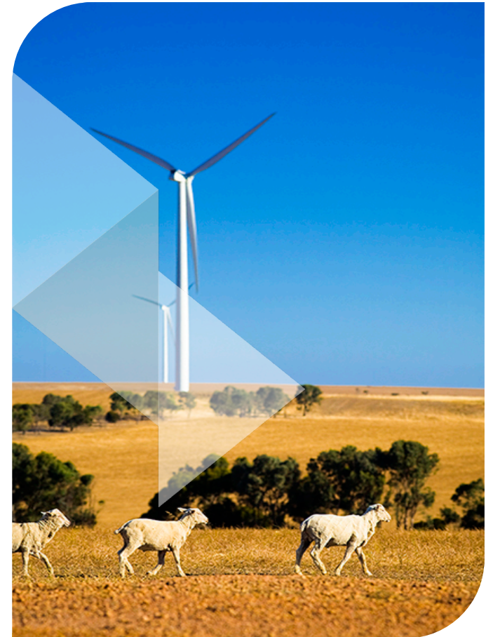
Alinta Wind Farm
