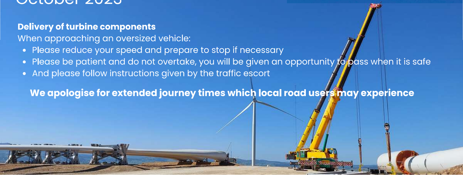
Turbine component deliveries for Turbine 36, Collector Group 1-West, 19 October 2023
